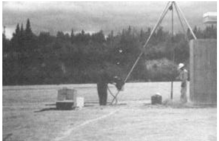
Installation of a monitoring well for a detailed site characterization in a Cree community.
