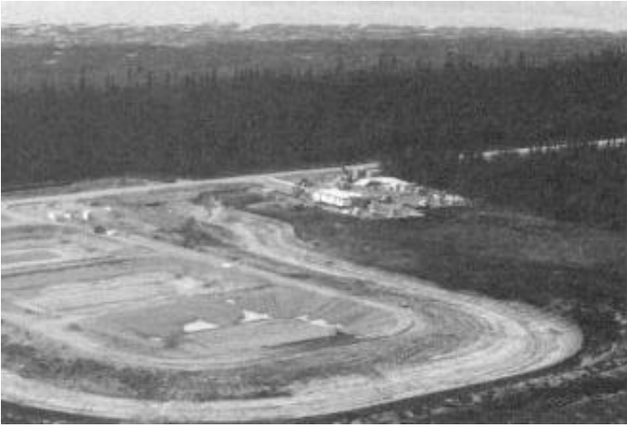
View of three aerated ponds used for sewage treatment in Waskaganish.
