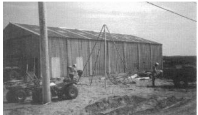
Monitoring groundwater quality in the Whapmagoostui municipal garage.
